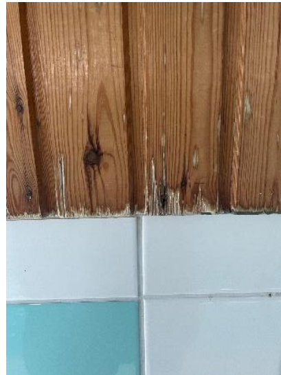
Fuktskadad panel
